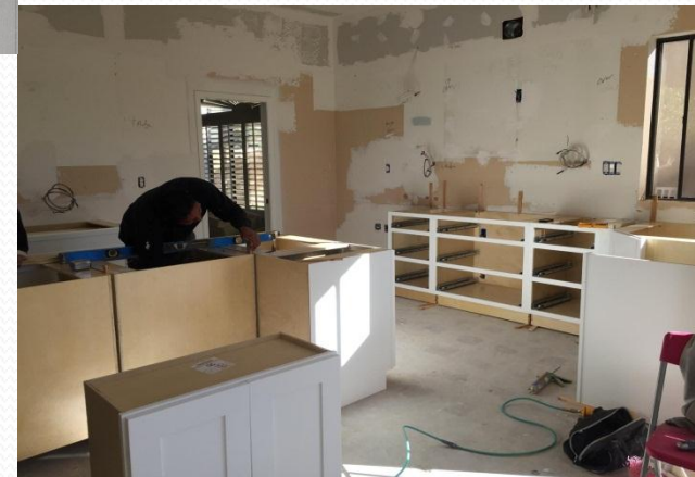
Construction of kitchen
